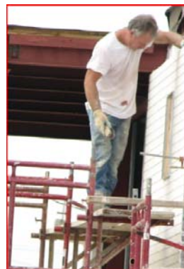
These workers are not protected from a leading edge fall.
