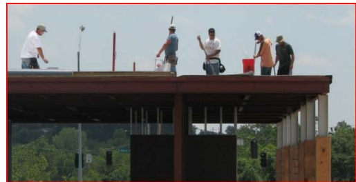
These workers are not protected from a leading edge fall.
