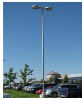
Make sure parking lot and security lights work.
