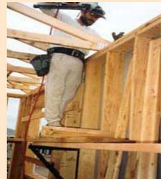
*Set up knee brace scaffolds and trusses from the inside of the wall.*
