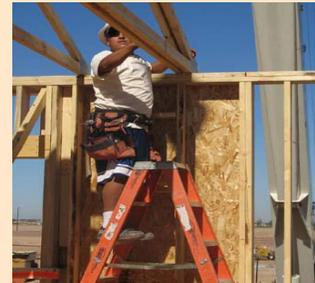
*Use ladders and set trusses from the inside of the wall.*
